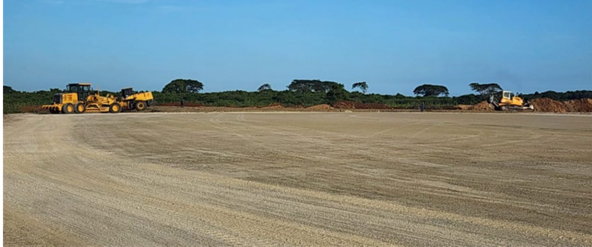
Figure 2 - Completed Pad 4 (Amistad-3)
