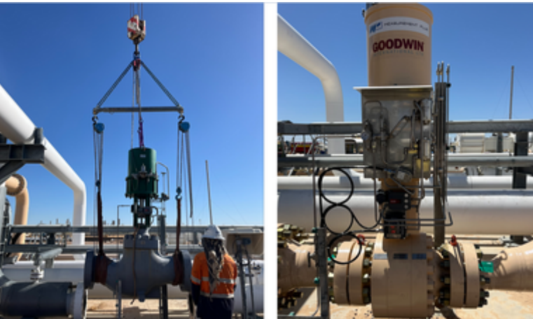
Installation of a new valve with a low-bleed digital valve controller at our Moomba hub.
