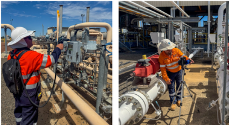
Our methane measurement campaigns apply international frameworks and approaches to detect and measure fugitive, vented, incomplete combustion, and non-routine methane emissions.
