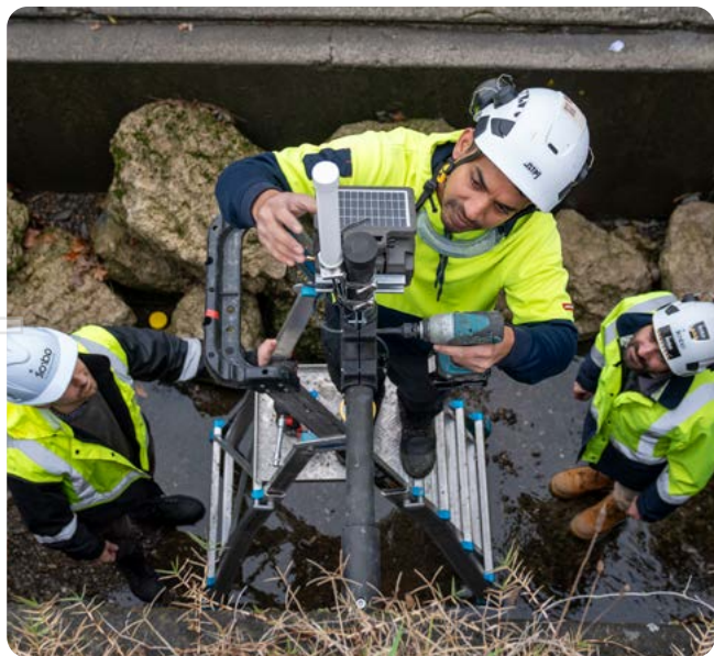
Technicians installing solar-powered sensors in Havelock North.
