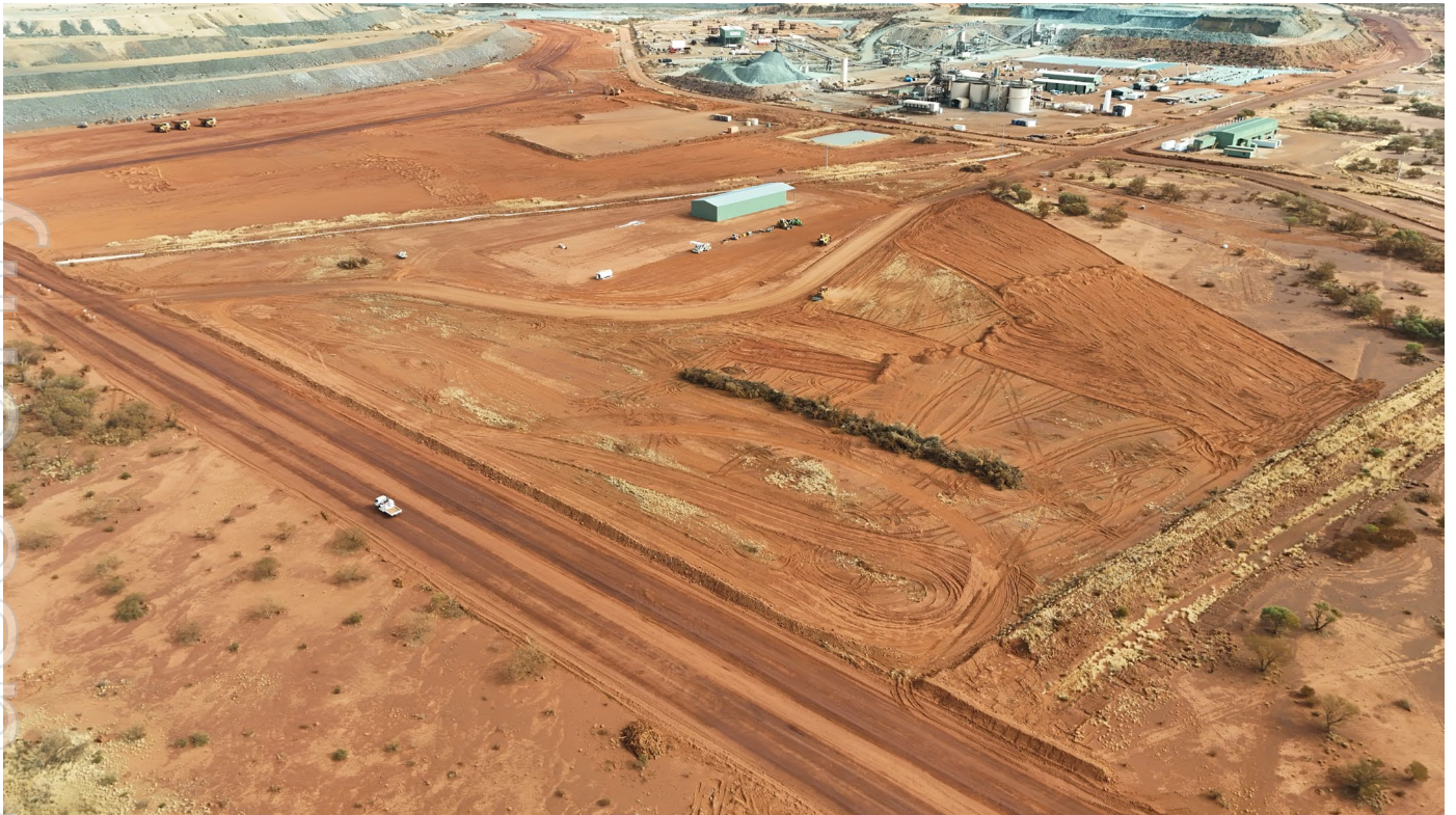
Karlawinda Expansion Project – Early Clearing Works
