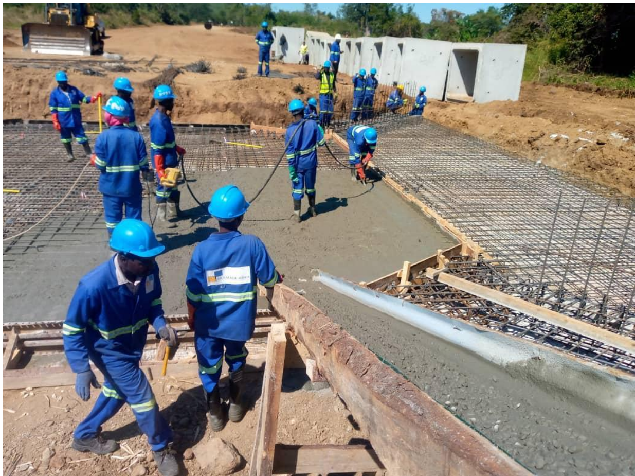
Figure 2. First concrete pour underway at Kangankunde, marking a major milestone in civil construction
