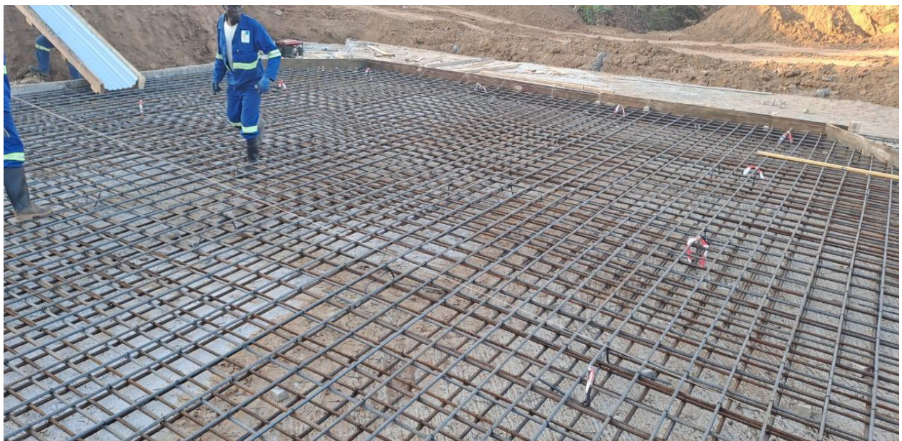
Figure 1. Rebar foundation work underway, setting the stage for the first major concrete pour at Kangankunde.
