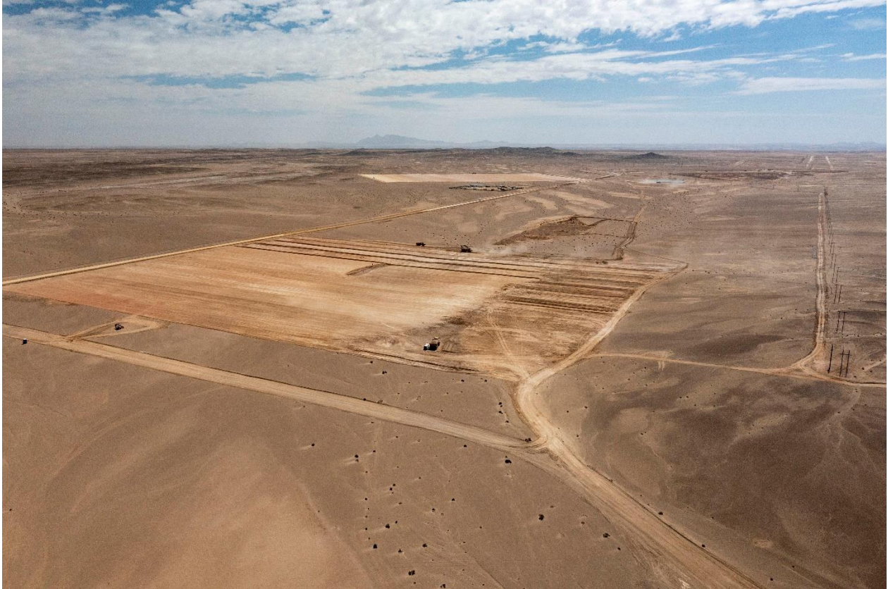
Figure 2: Clearing in preparation for heap leach pads 1 and 2.
