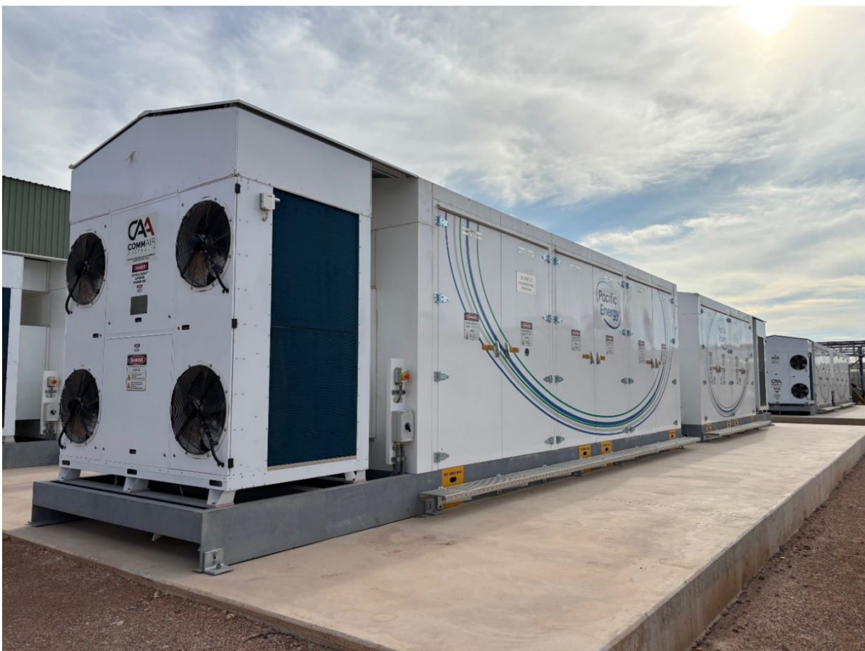
Figure 1: The Pilgangoora Operation lithium powered battery energy storage system.
