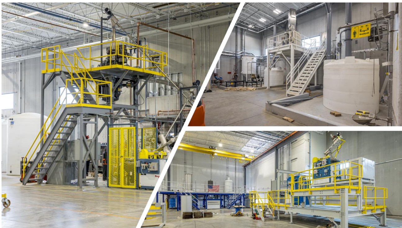
Figure 2: Ancillary Equipment and Utilities Installation
