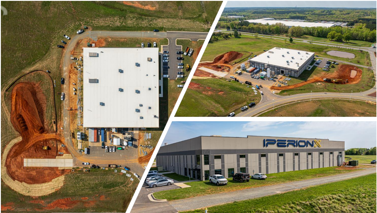
Figure 1: Titanium Production Facility, location of the HAMR furnace operations
