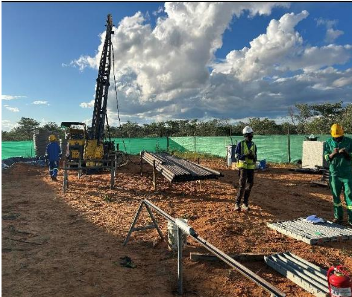
Figure 3: Drill rig on site at Fiesta recovering core in hole 25FIEDD025
