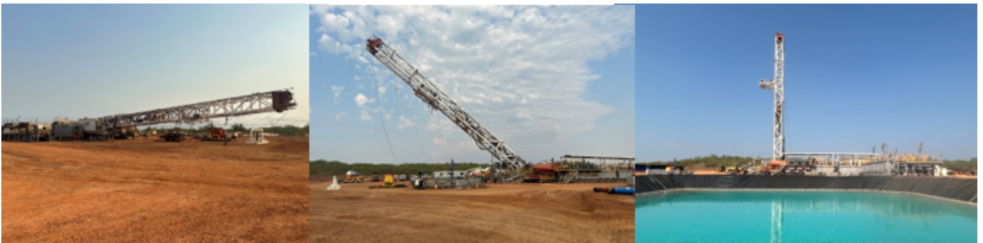
Ensign Rig Being Mobilised at C-5H
