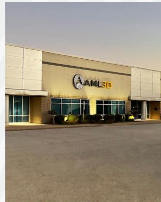
AML3D Stow Technical Facility
