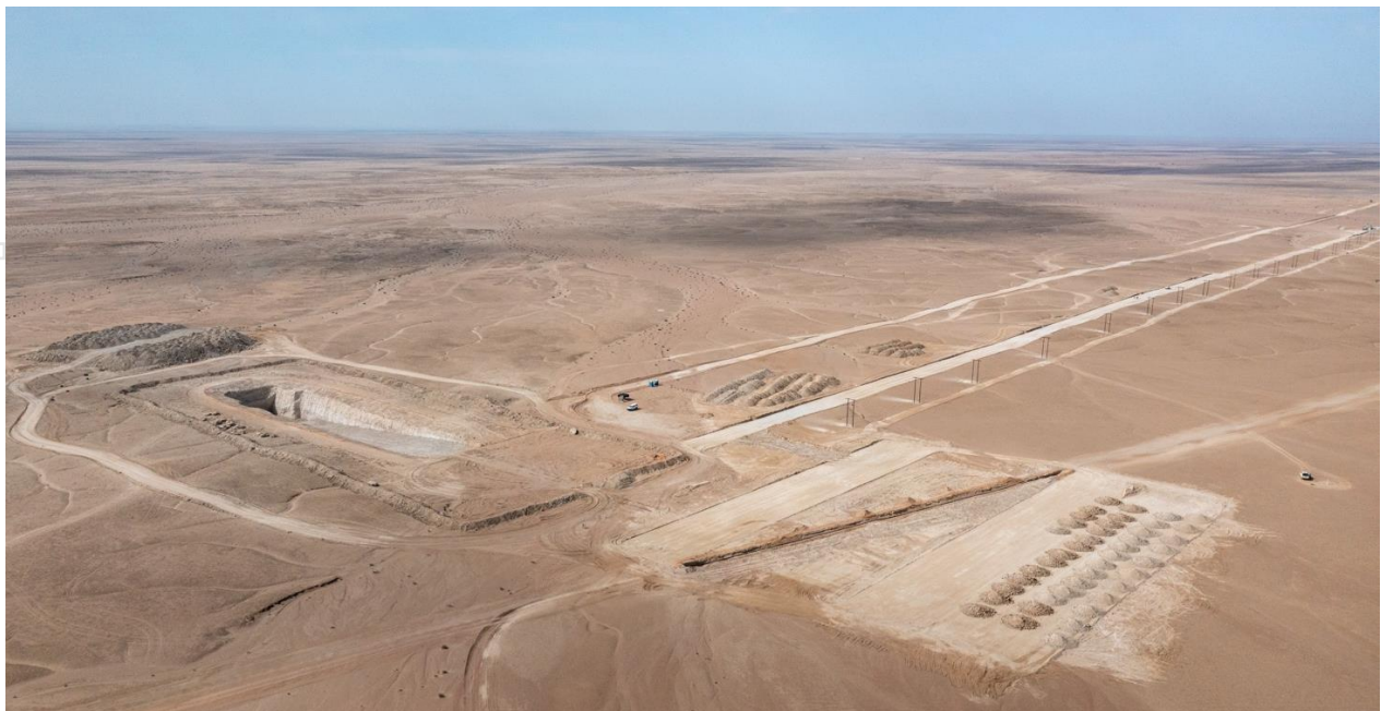
Figure 1: Significant progress continues on bulk earthworks at Etango, a key enabler of future construction and development activities. The primary crusher has been fully excavated and its dimensions confirmed, while work advances on the permanent road and conveyor belt line to the secondary and tertiary crushing areas.
