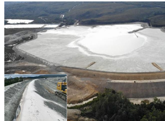
Henty TSF and Jan 2025 works (inset)
