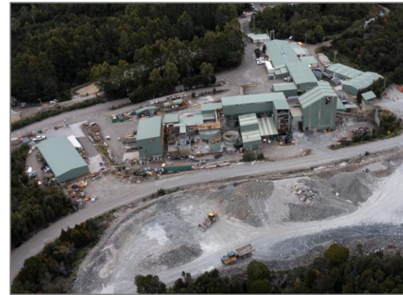
300ktpa CIL Plant & Administration Complex
