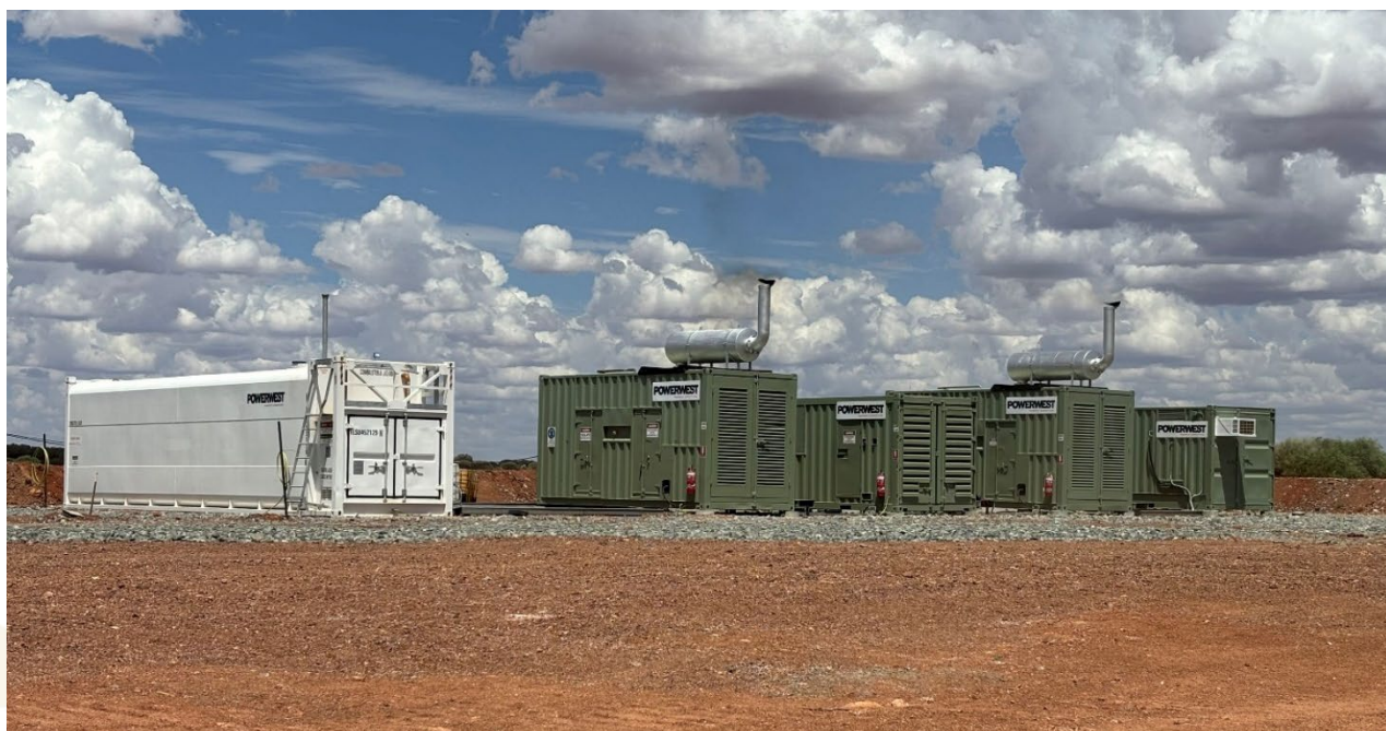
Figure 3: 2.8MW diesel power station recently commissioned
