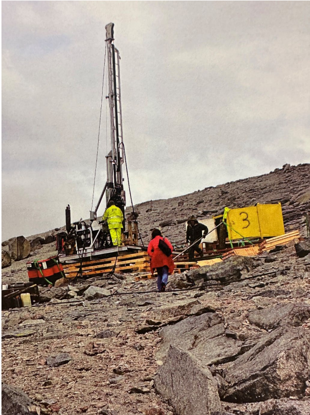
Figure 5 Diamond drilling 2013 over eudialyte surface outcrop (in foreground) over the Fjord MRE Zone
