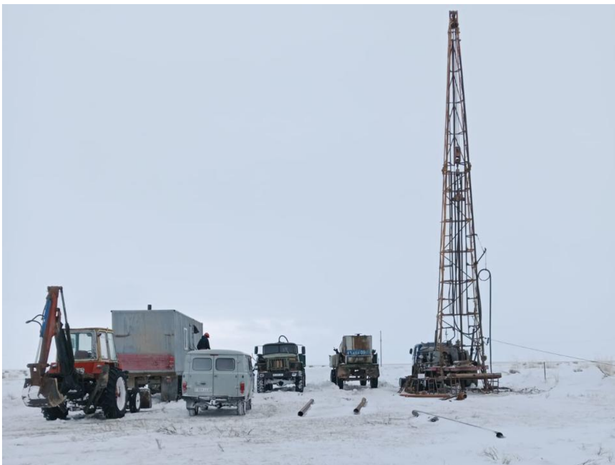
Figure 1 – Water bore drilling underway in the Sherubainura River Aquifer
