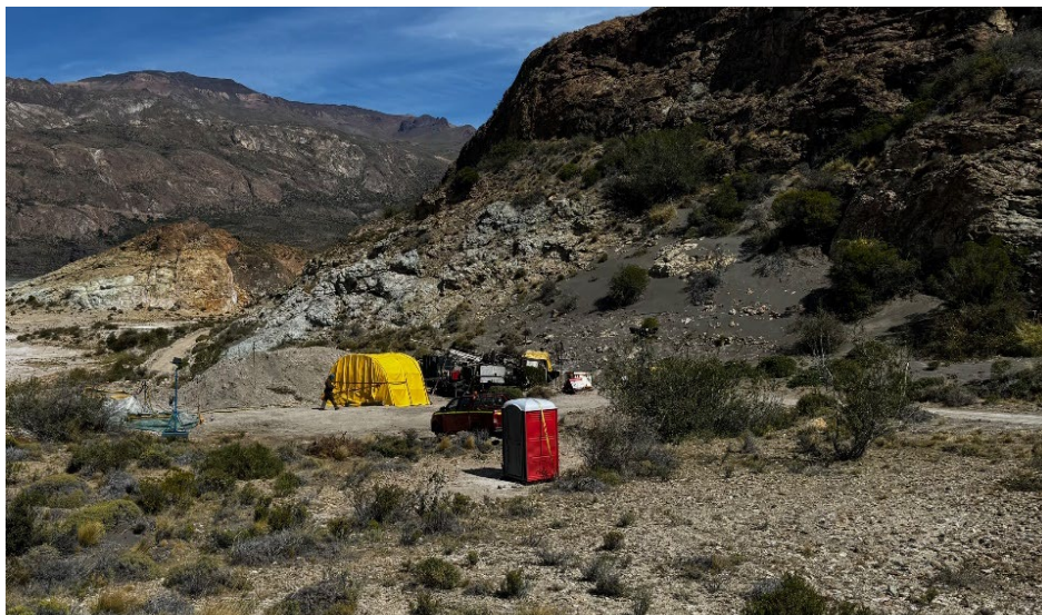
Figure 1. Coyita North drill platform testing the northern shoot.
