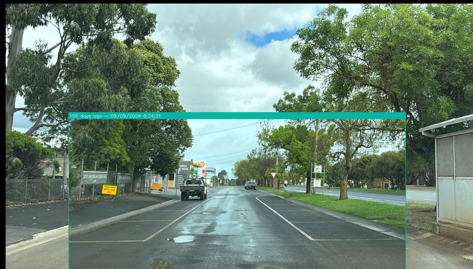
< Previous inspection #1 at the same location
