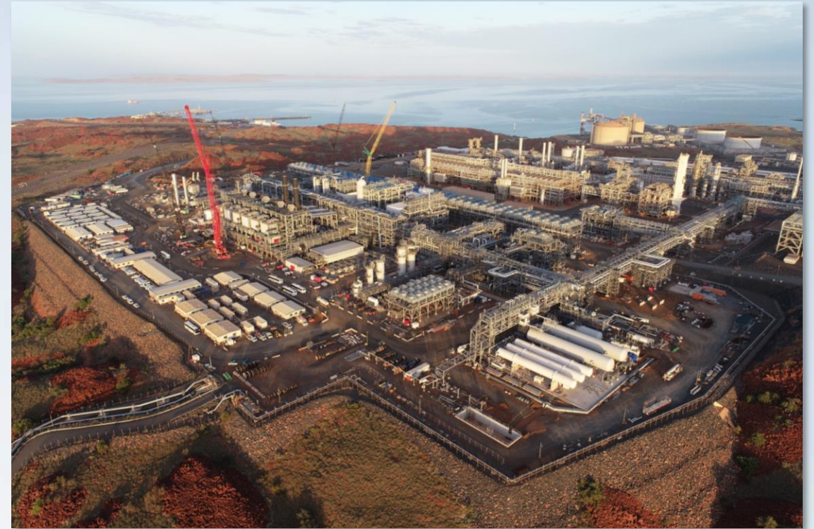
Pluto Train 2 construction progress
