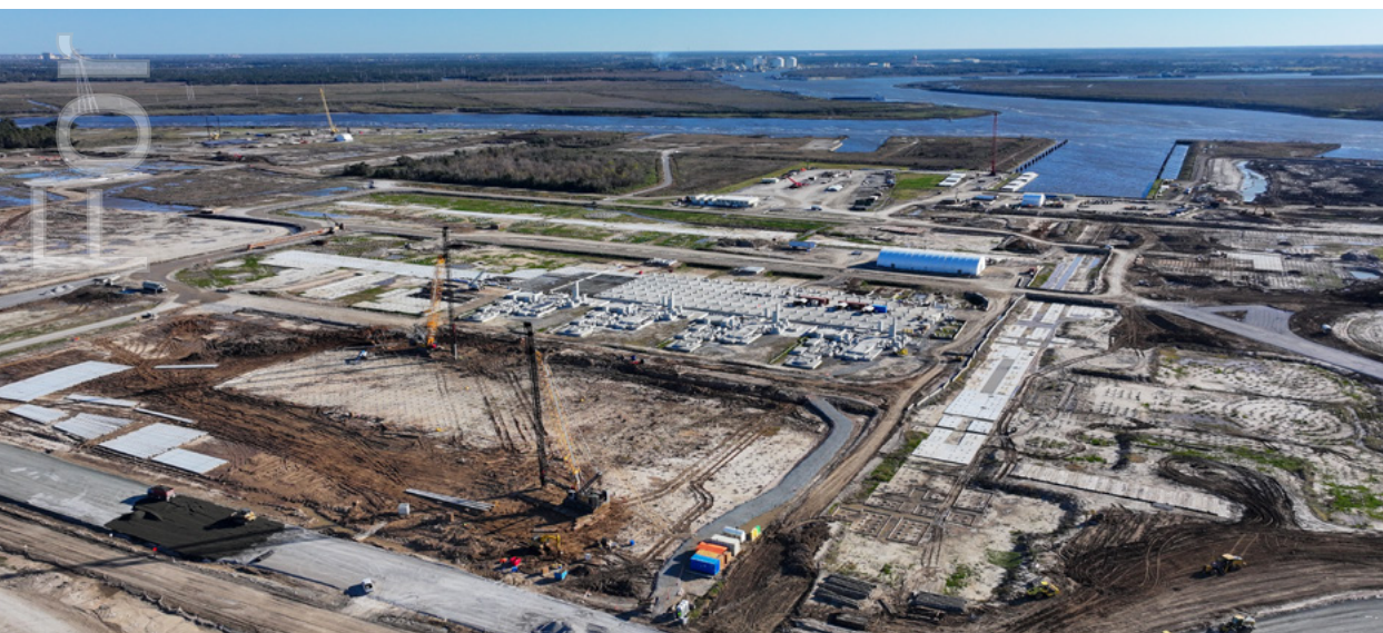
Woodside Louisiana LNG development, January 2025
