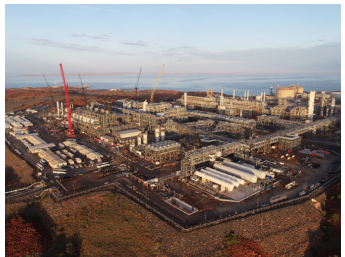
Pluto Train 2 construction progress, Western Australia, December 2024
