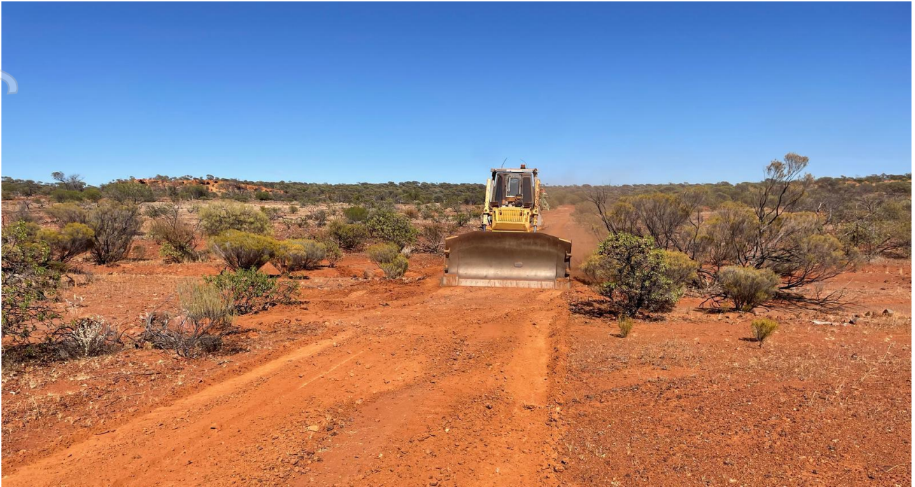
Figure 1: Site works commencing for March drilling program
