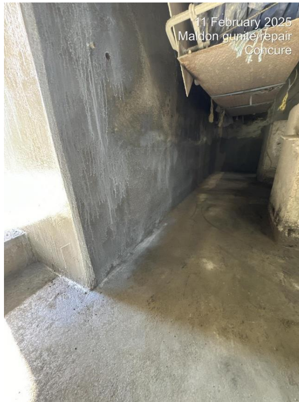
Figure 8: Photo of a section of the replacement high strength concrete foundation of the processing plant, that supports the ball mill
