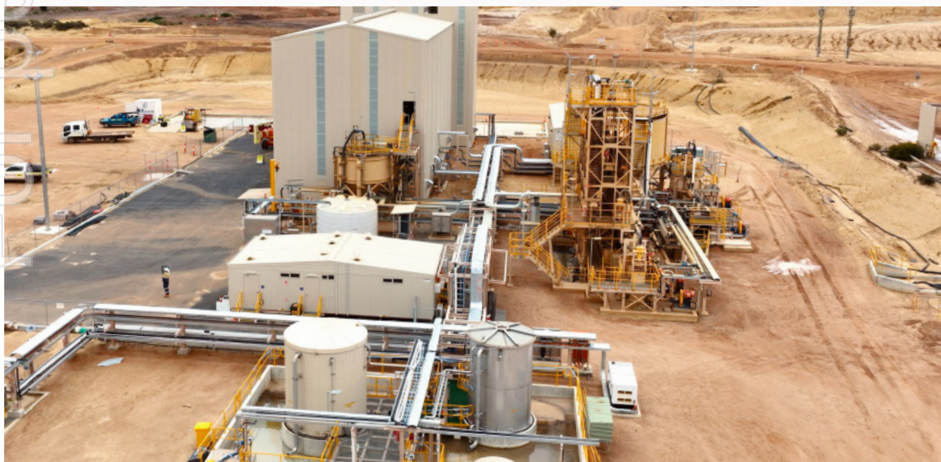
Beneficiation plant at Eneabba.
