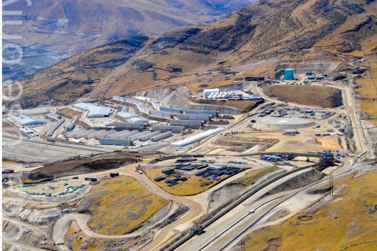
Figure 7: Image of mine and infrastructure at Las Bambas Mine – Peru's 3 rd largest copper deposit accounting for 2% of global production. Located 60km along strike of Venatica on the same structural trend and sharing the same host geology and key deposit feature positioned on the contact margin of the Andahuaylas-Yauri Intrusive Batholith. 1,2
