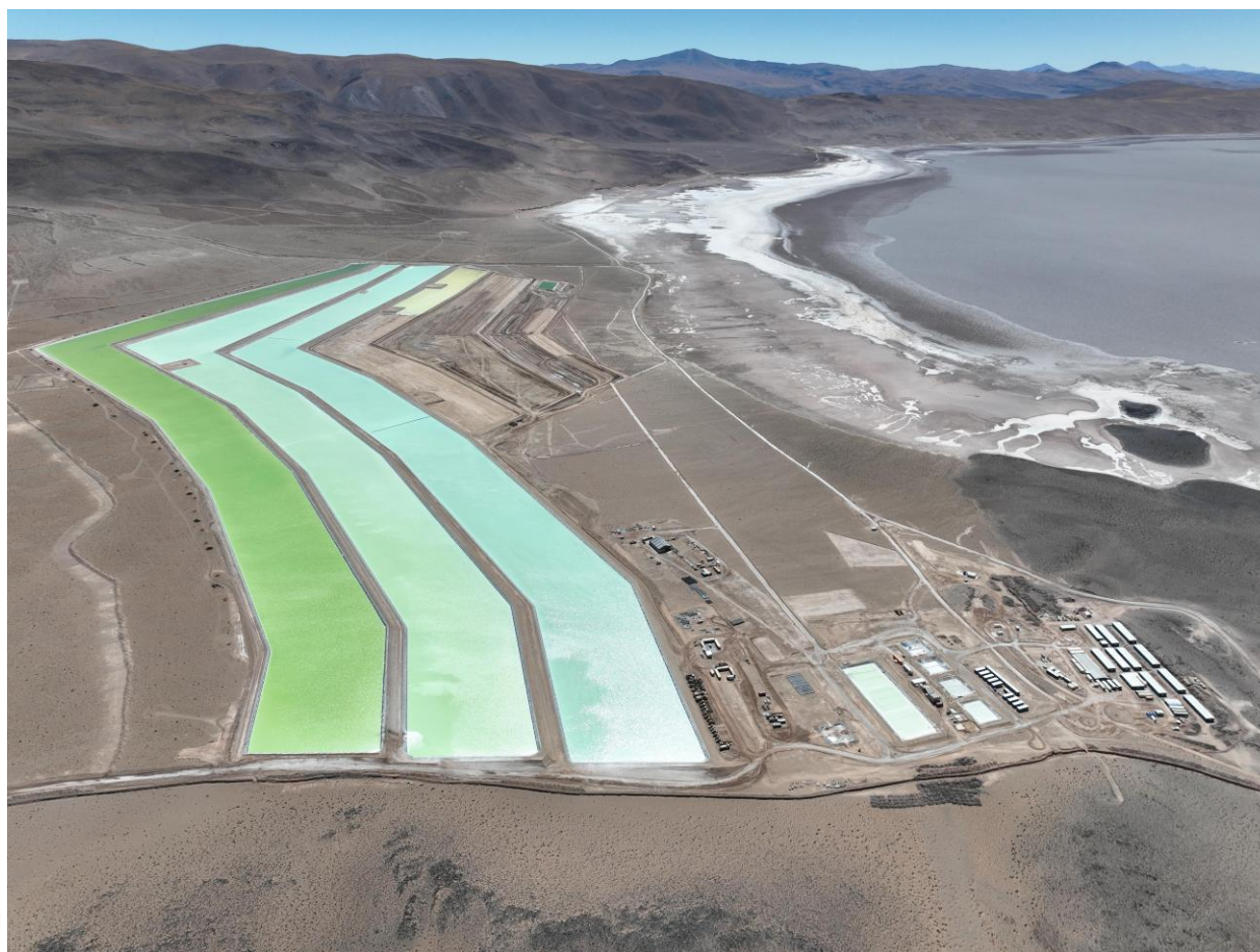
Figure 3 – General Overview of HMW Site
