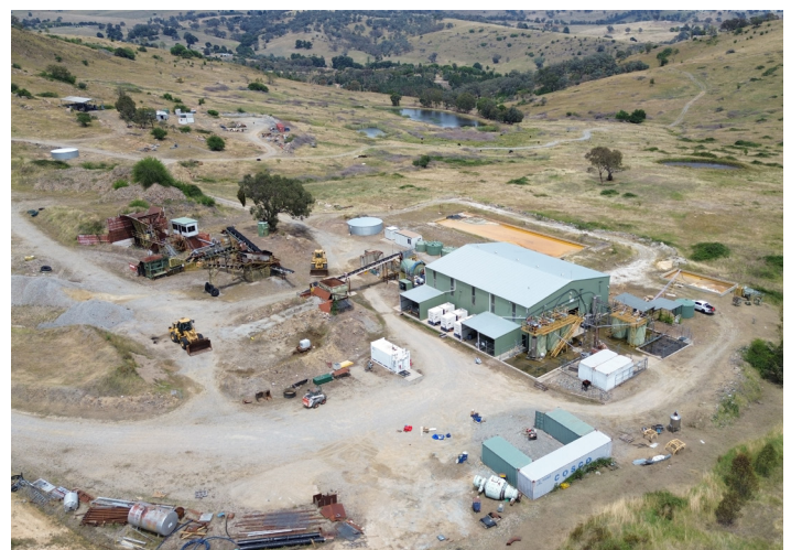
Above: Drone overview of the plant area before upgrades were completed
