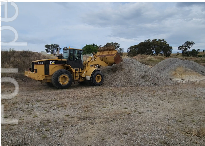
Above: Loader after being repaired on site.
