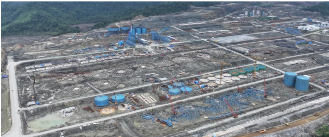
ENC HPAL construction progressing well
