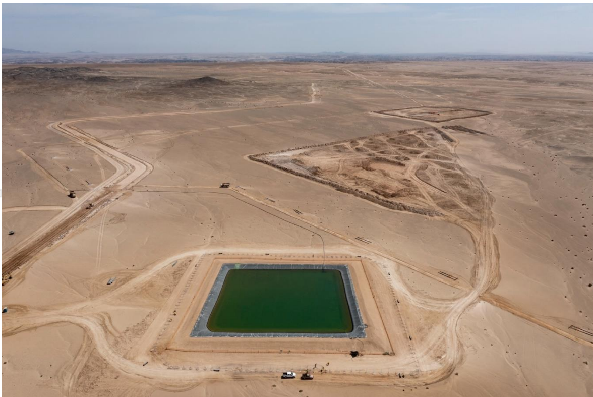
Figure 1: Completed construction water storage dam
