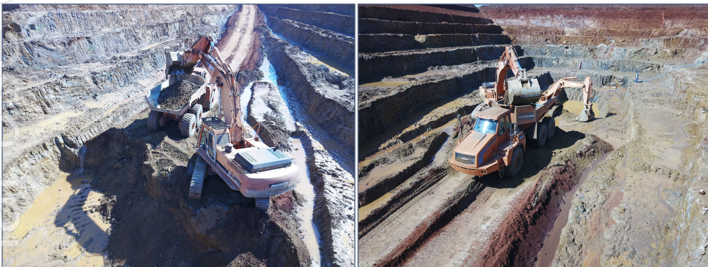
Figures 7 & 8: Simple excavator fleet mining the test pit
