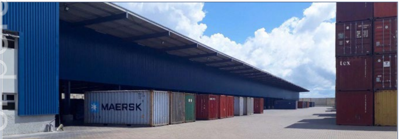
Figure 23: Grindrod's back of port facility at Nacala Port
