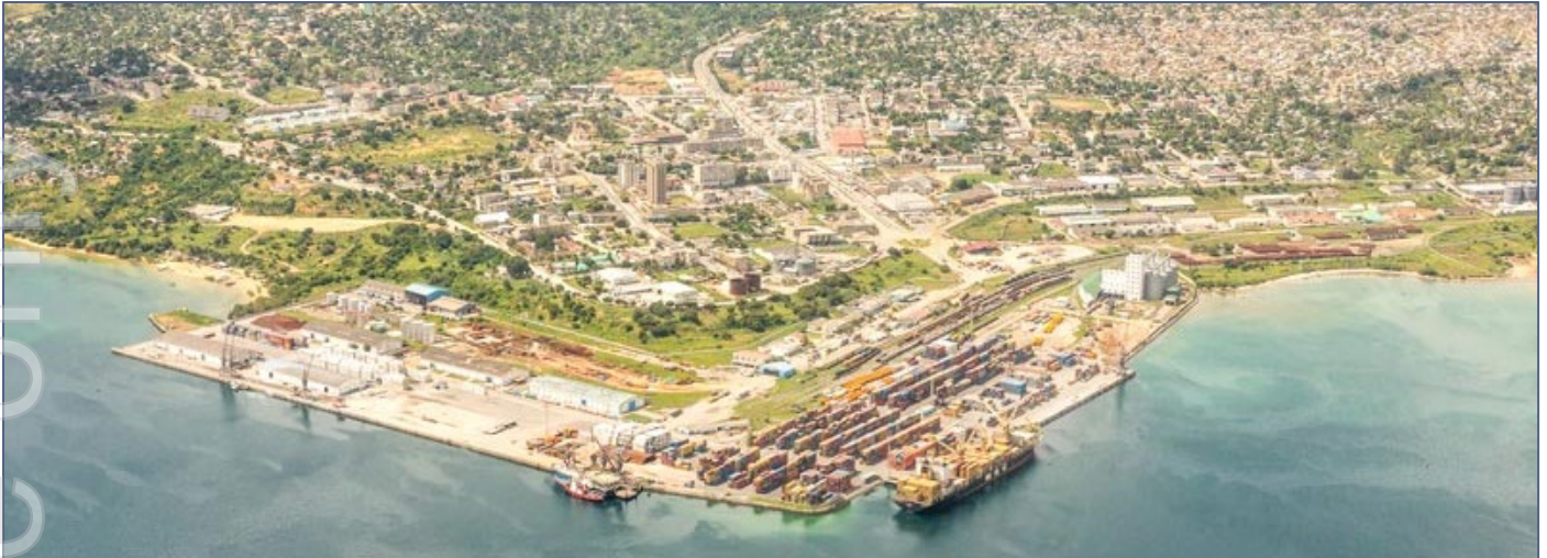
Figure 24: Port of Nacala, Mozambique
