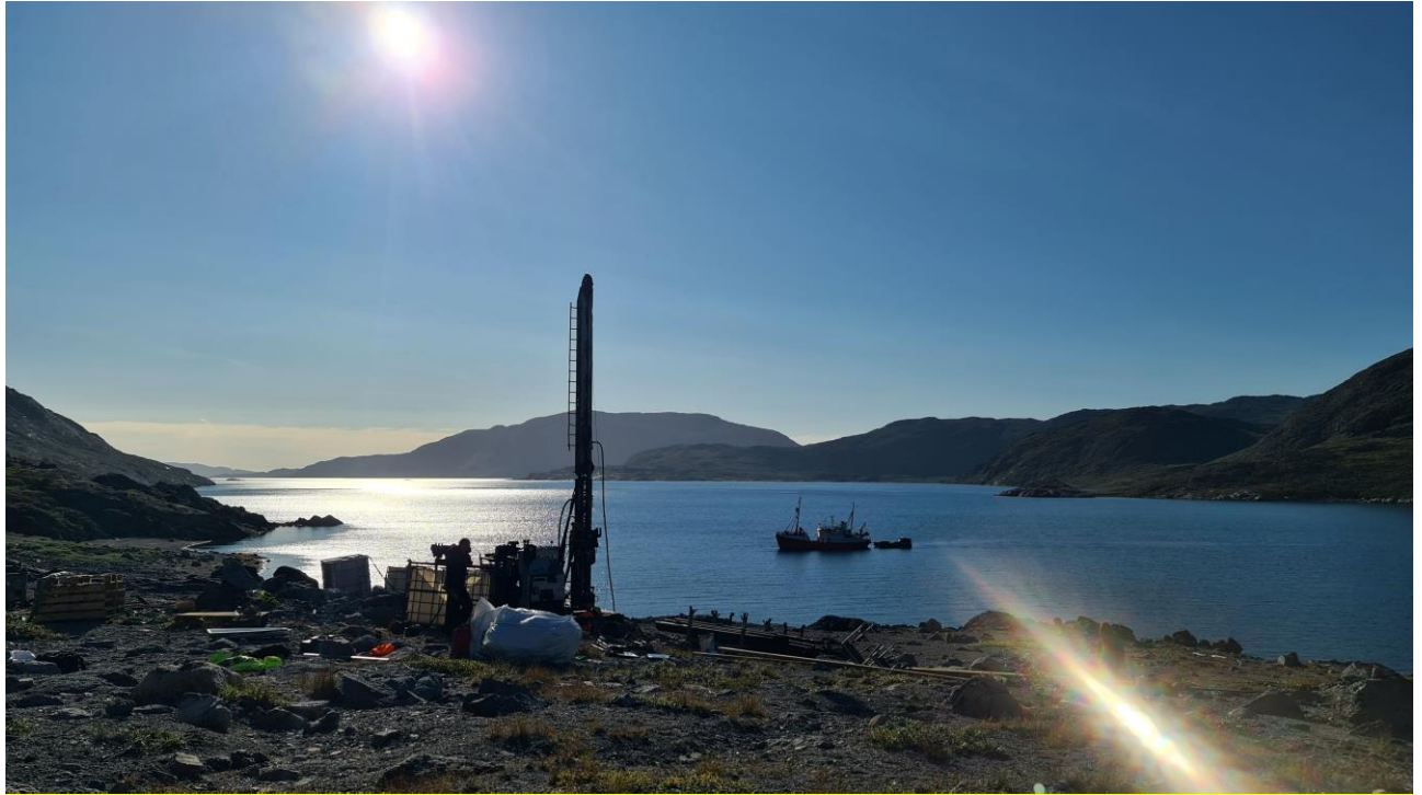
Photo 1. Drill rig commences operations at the Tanbreez Project in Greenland.
