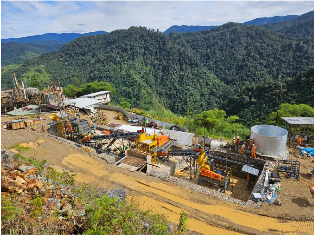
APT modular gravity plant installation, Dec 2024
