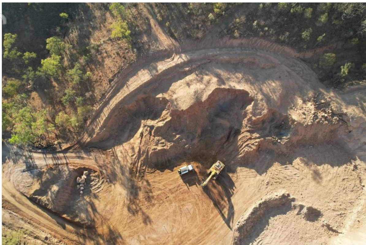
Mining Pit 4 December 2023
