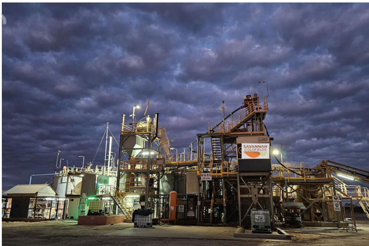
Georgetown Processing Plant
