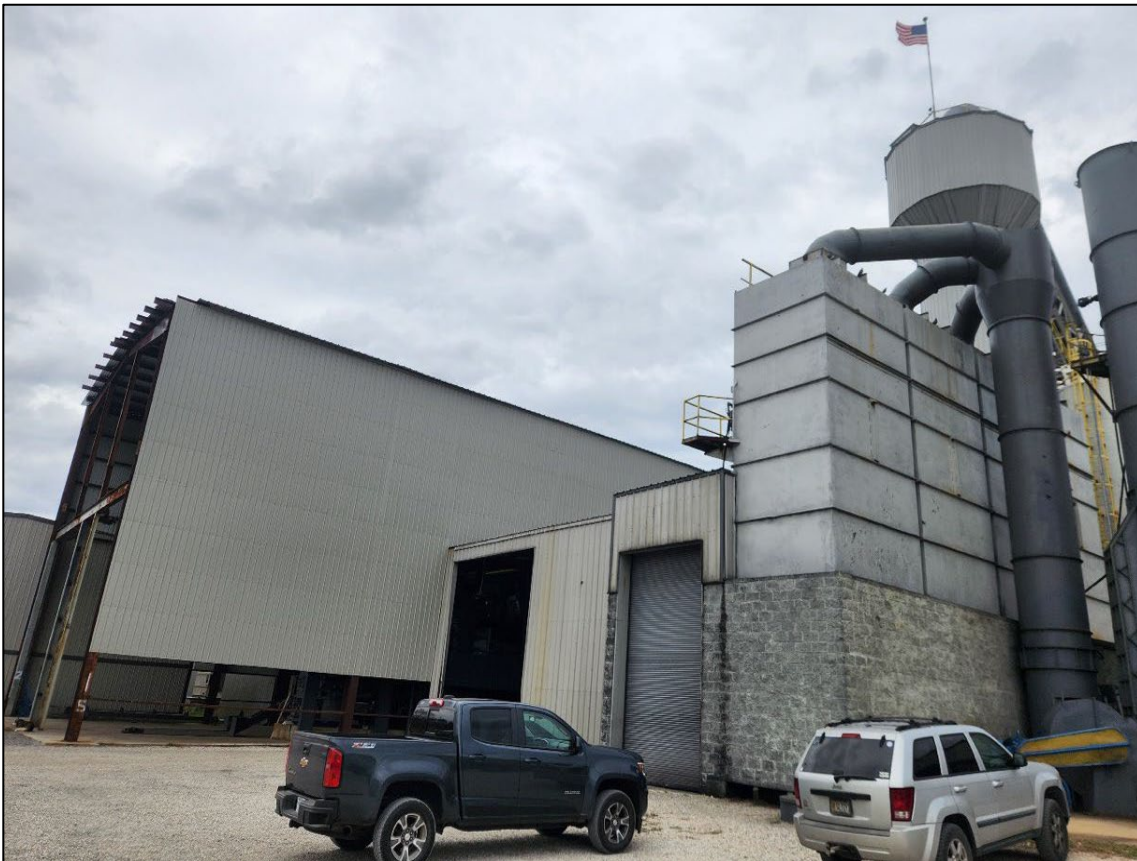
Image 1: Front view of the Kentucky Plant, highlighting its conversion to a high-capacity Activate Carbon production facility.
