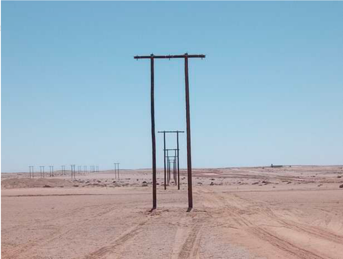
Figure 2: 33kV powerlines H-pole support structures being installed
