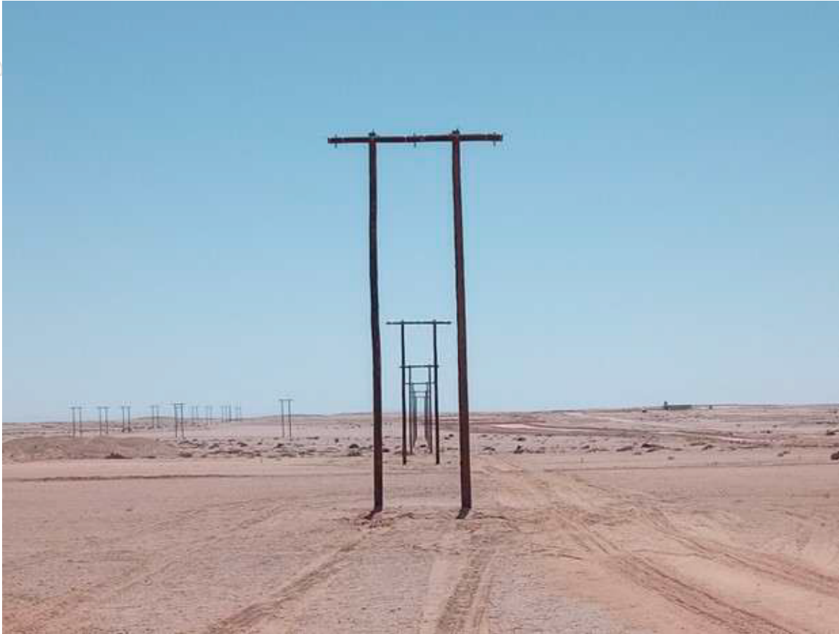
Figure 2: 33kV powerlines H-pole support structures being installed
