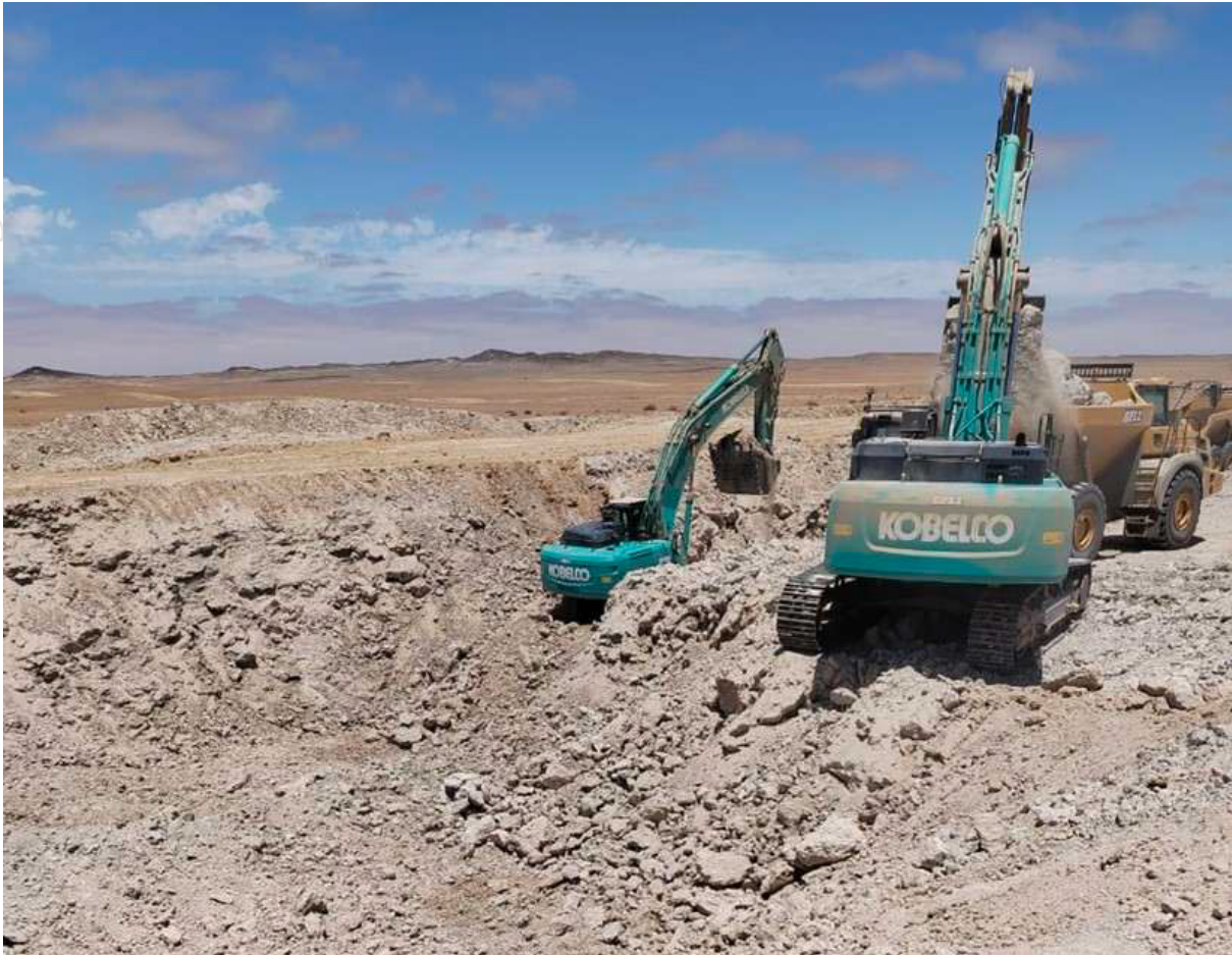
Figure 4: Excavation of primary box cut post blasting
