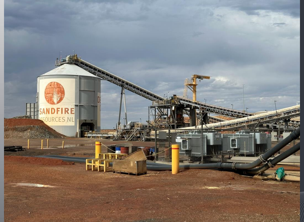
Figure: DeGrussa Process Plant
