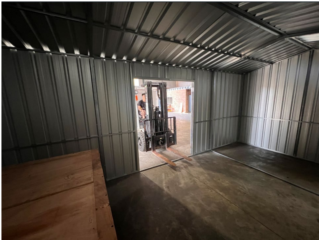
Figure 1: Internal view of Clean Room 1
