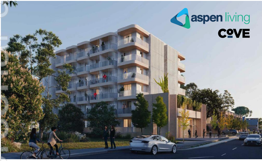
Aspen CoVE Apartment Complex
