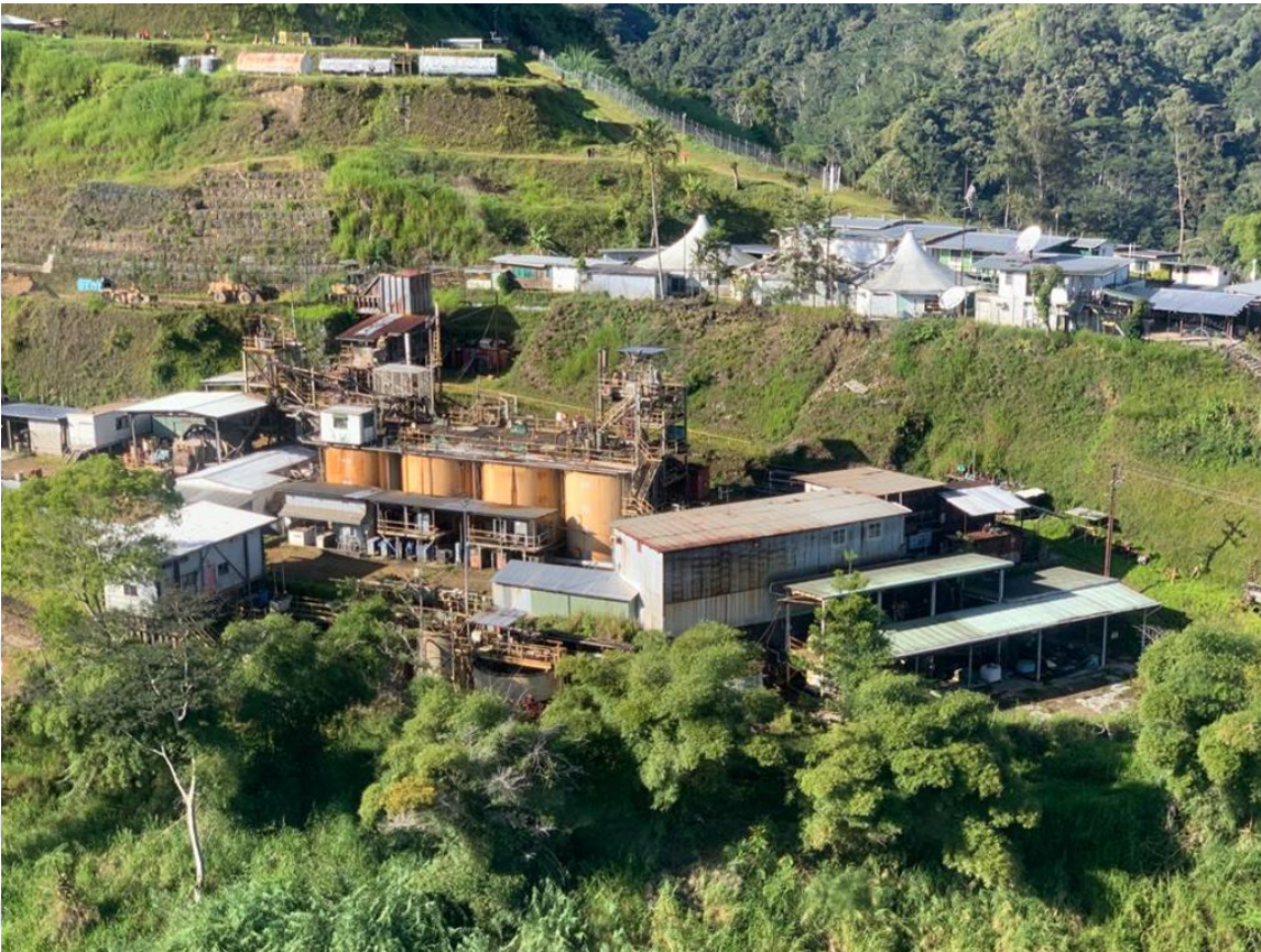
Infrastructure in place
