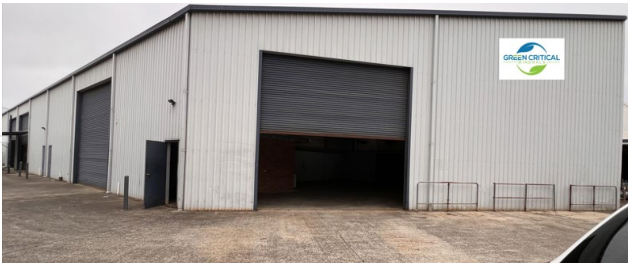
Figure 1 Green Critical Minerals VHD Technology Industrial Facility.
