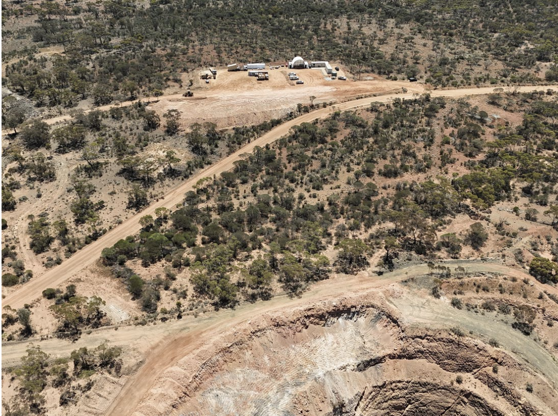
Figure 2: Aerial view of Offices, Workshop and Laydown in background of Newhaven Pit
