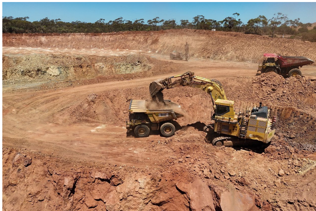
Figure 3: 200 tonne excavator loading truck in Newhaven Pit 405m RL
