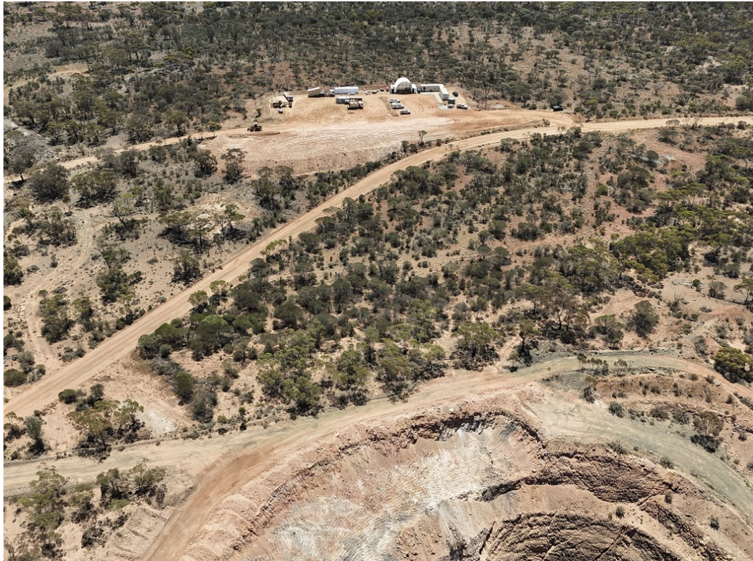
Figure 2: Aerial view of Offices, Workshop and Laydown in background of Newhaven Pit
