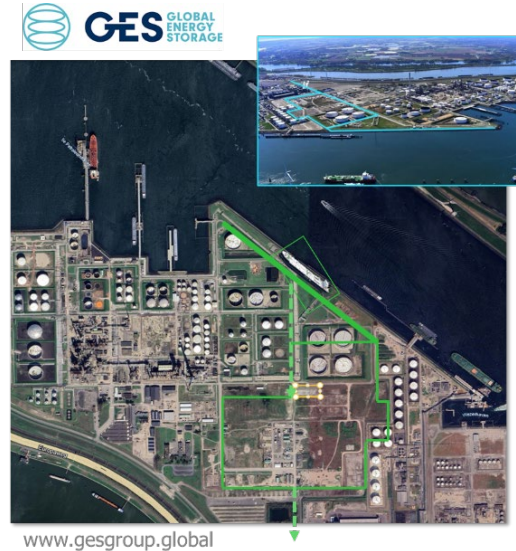
GES Terminal Site at the Port of Rotterdam, Netherlands
