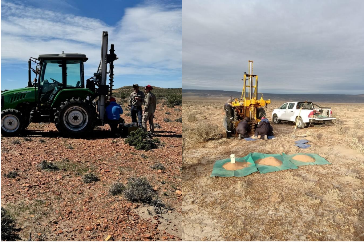
Figure 4 : The two auger drill rigs at Sierra Cuadrada testing for visible uranium on a broad spaced grid to enable the Company to focus on priority areas for future trenching.
