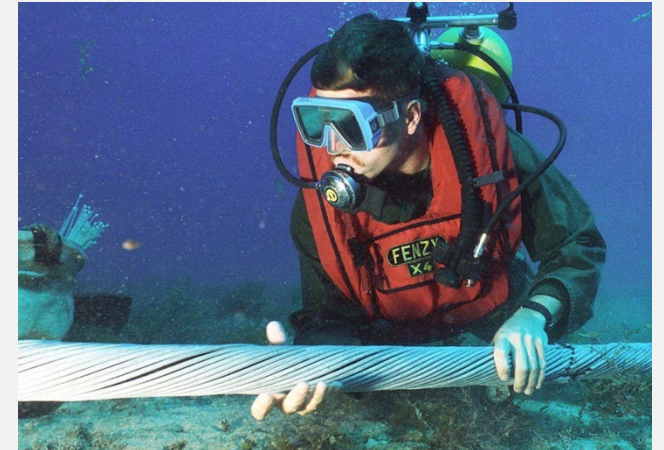
Monitoring of subsea telco cables
