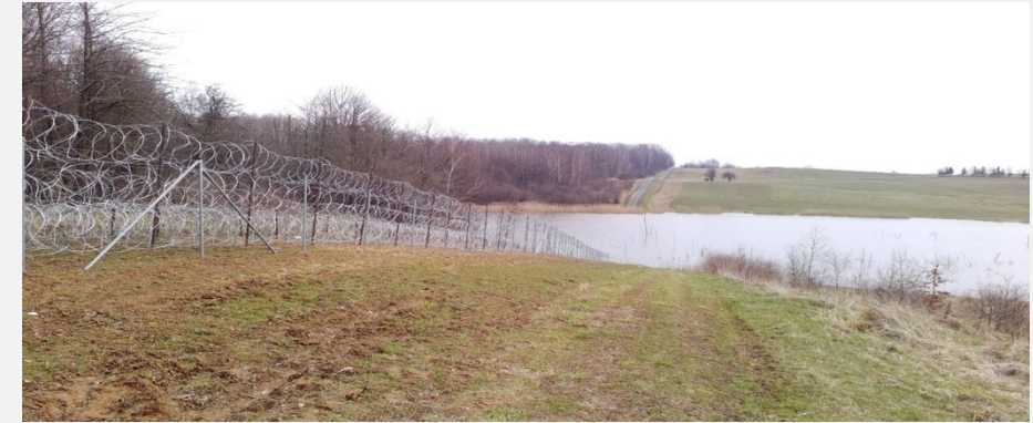
Fence along border
