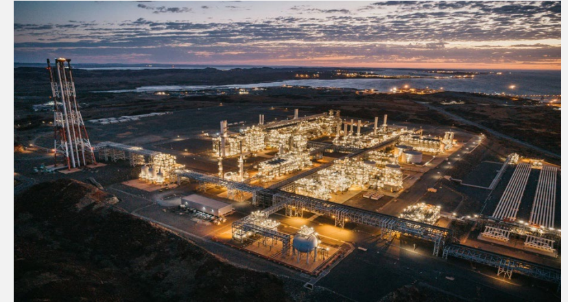
Major facility installed PIDS
