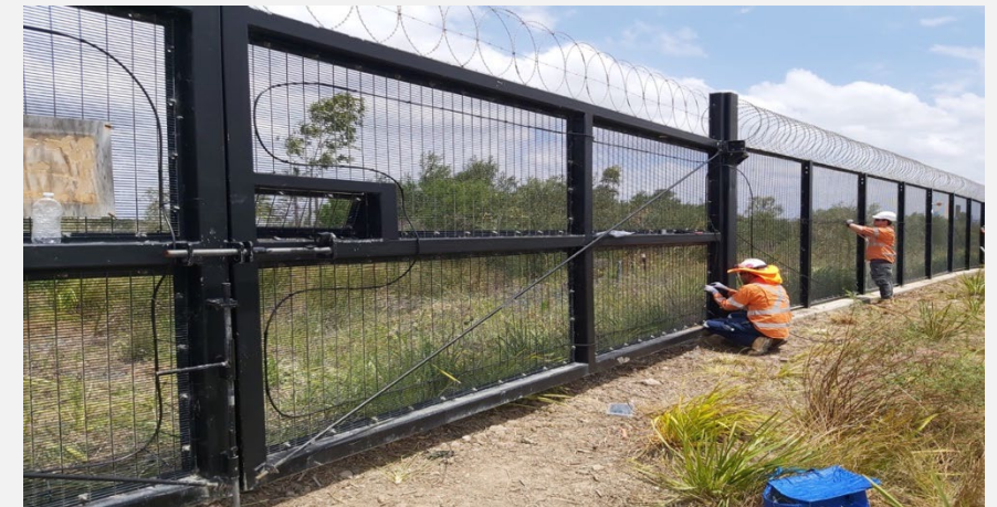
Security fence for rail corridor
