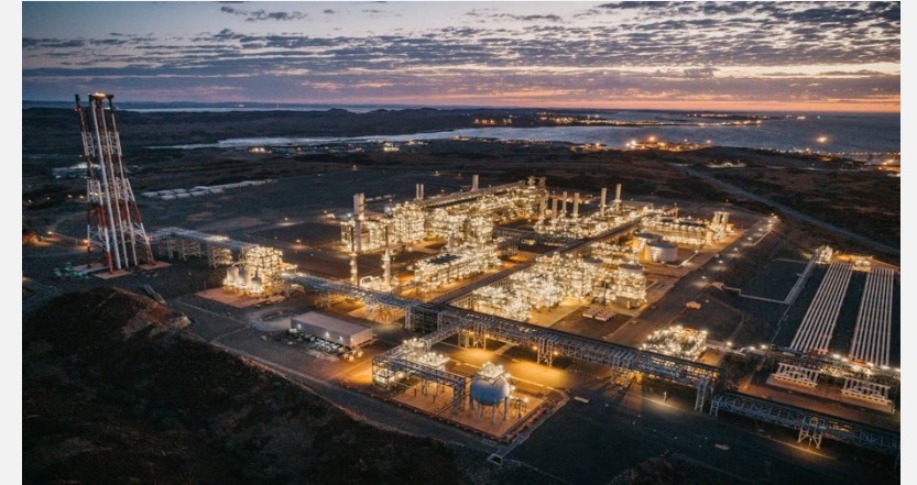
Major facility installed PIDS
