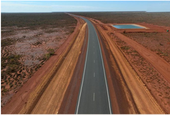
Onslow Haul Road West
