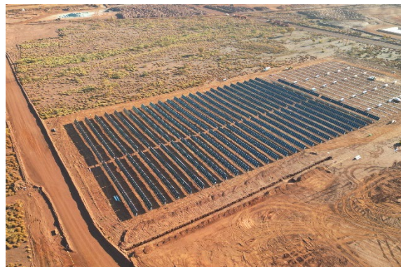
Solar array under construction at Ken's Bore
