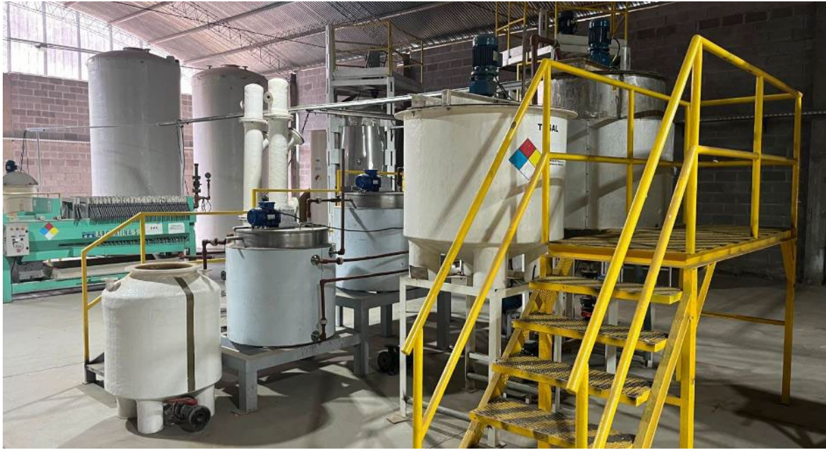
Figure 5: 250tpa Lithium Carbonate Plant at Pursuit's purpose facility in Salta, Argentina
