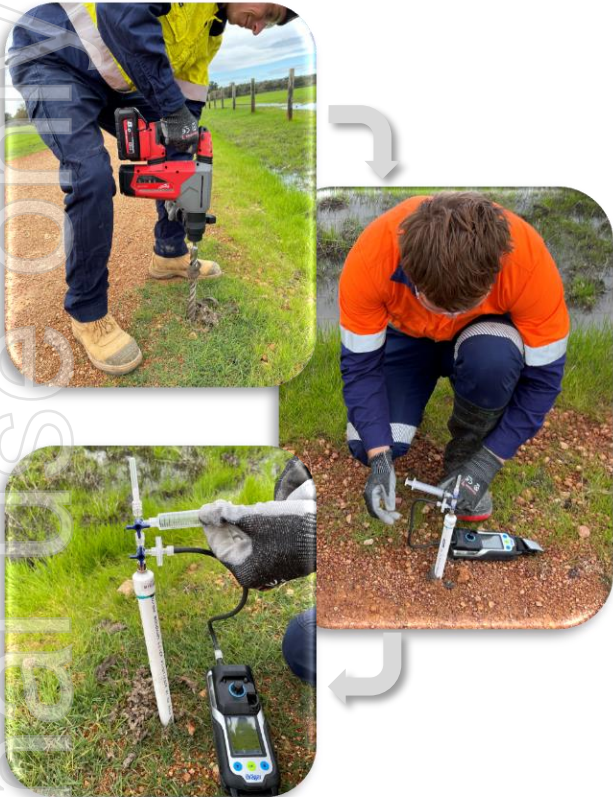
Spot soil gas sampling equipment
