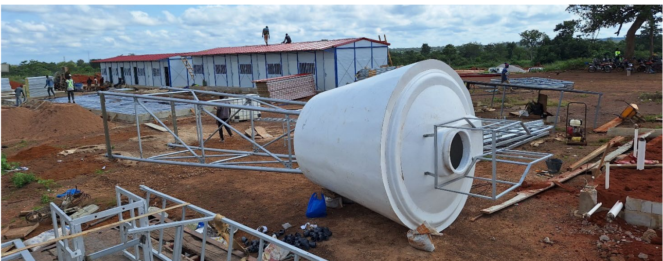
Figure 7 Boundiali central exploration camp (Dougoujin Camp) in construction
