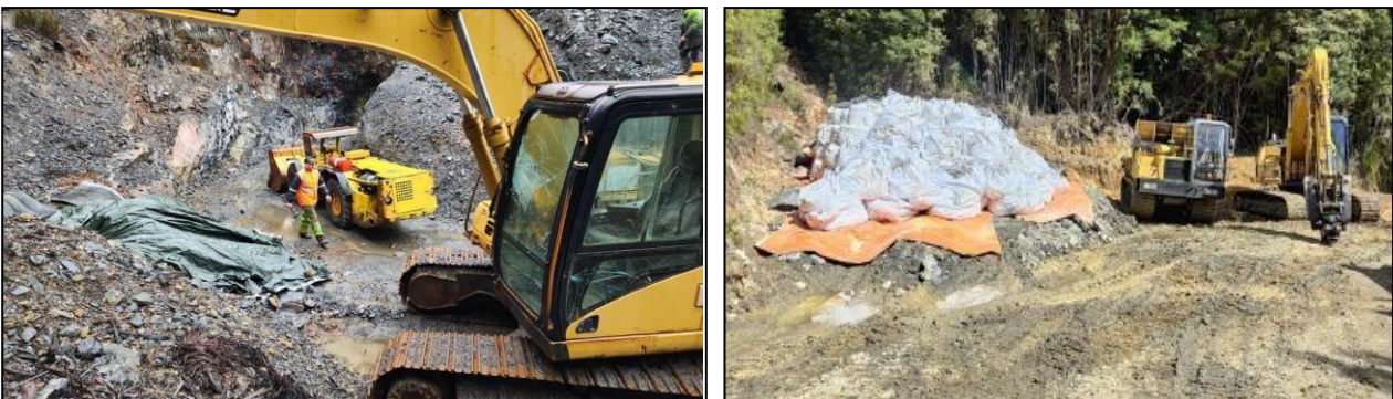
Figure 9. Montezuma Antimony Project mining equipment and stockpiled development mineralisation, potentially DSO.
