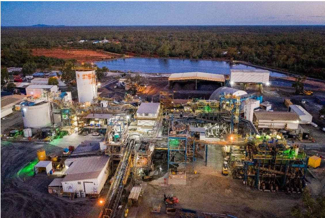
Figure 1: Peak processing plant, showing leach (left), comminution (centre), flotation (right), and filtration (back)
